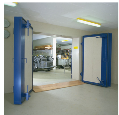
Concreted door in use
